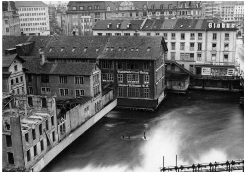
Six years later, in 1949, the demolition of the buildings downstream of the Mühlestege began. (In the background the old Globus building can be seen.)
