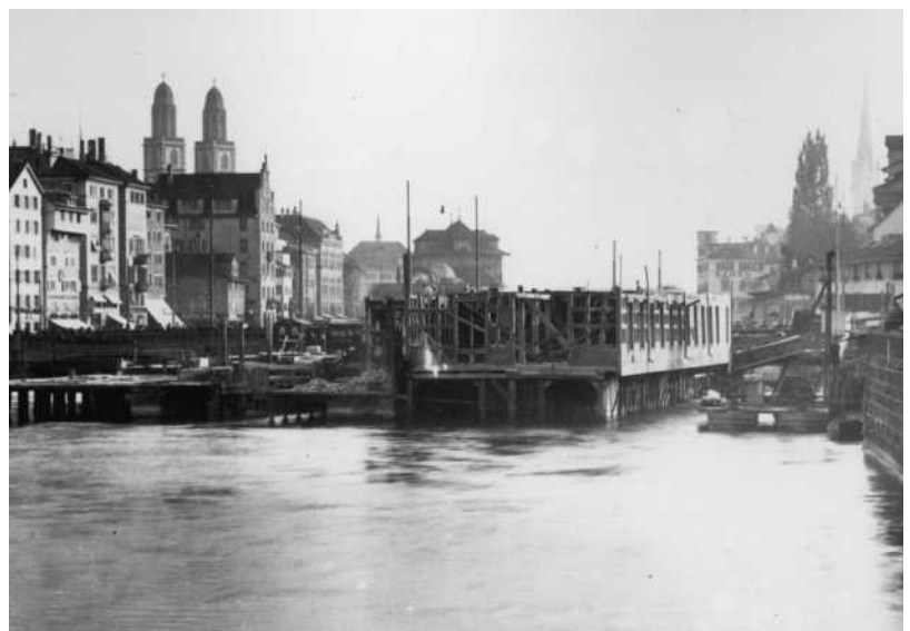
Due to new urban policies and an improvement of the channel to Lake Zurich, in 1943 the buildings that inhabited the Limmat River on the upper part of the Mühlesteig bridge were demolished.
